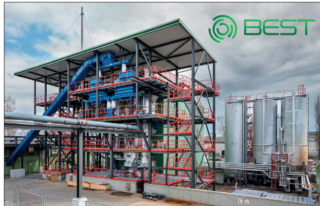
Left: Methanization fluidized bed of TU Vienna.
